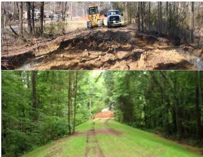
Top: Excavation of PAH-contaminated soil and ballast material. Bottom: Site restoration of Off-Base portions of rail spur.
